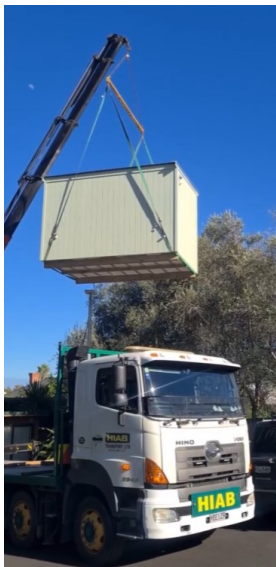
The new counselling room getting installed by Hiab crane!
